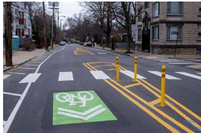
Green Back Shared Lane Markings
